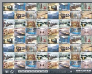
central monitoring system (CMS)
